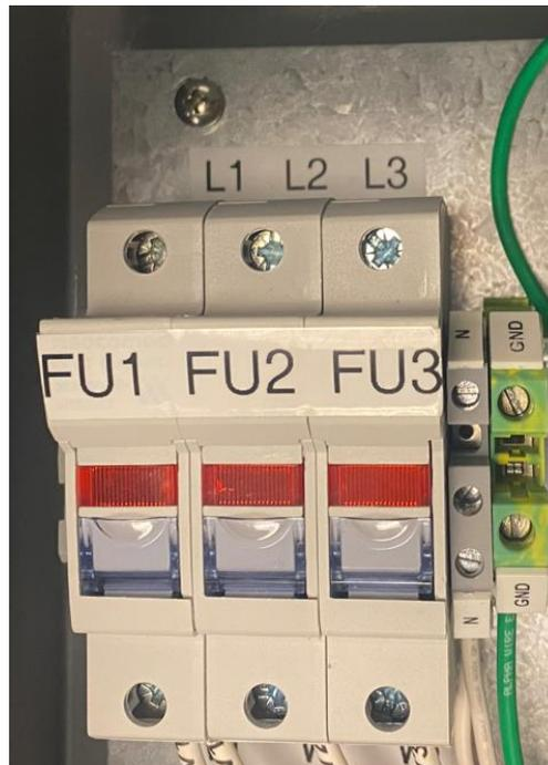
**Figure 3: Wire the voltage based on the labeled fuse holders (note that the fuse holders are empty).**
