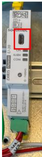
Figure 4: The micro USB port on the DIRIS Digiware U-30
