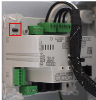
Figure 6: The micro USB port on the DIRIS A-40.
