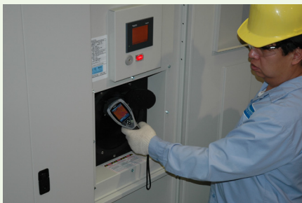
Technician scans the interior of a Powersmiths Energy Station™ PDU through the Rotatable IR Port with recessed mount as part of a preventative maintenance program.
